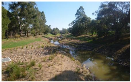
The Redevelopment of the Dandenong creek between HE Parker reserve and the Railway Bridge towards Bayswater called 'daylighting' involved the removal of the underground pipes that channel the creek water through this section. The original creek had been turned into a flood basin to prevent floods as residential properties were developed along the creek.
